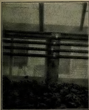
14.—Fastening pipes to posts by tin clips.
